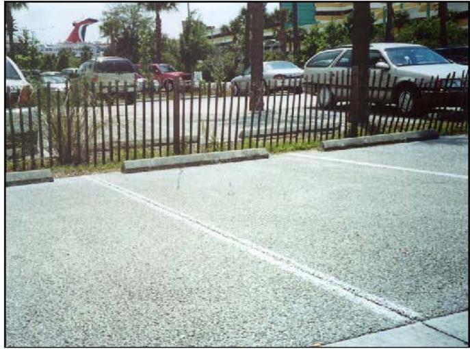
**Figure 2.2.24-3 Typical Porous Concrete System Applications**
