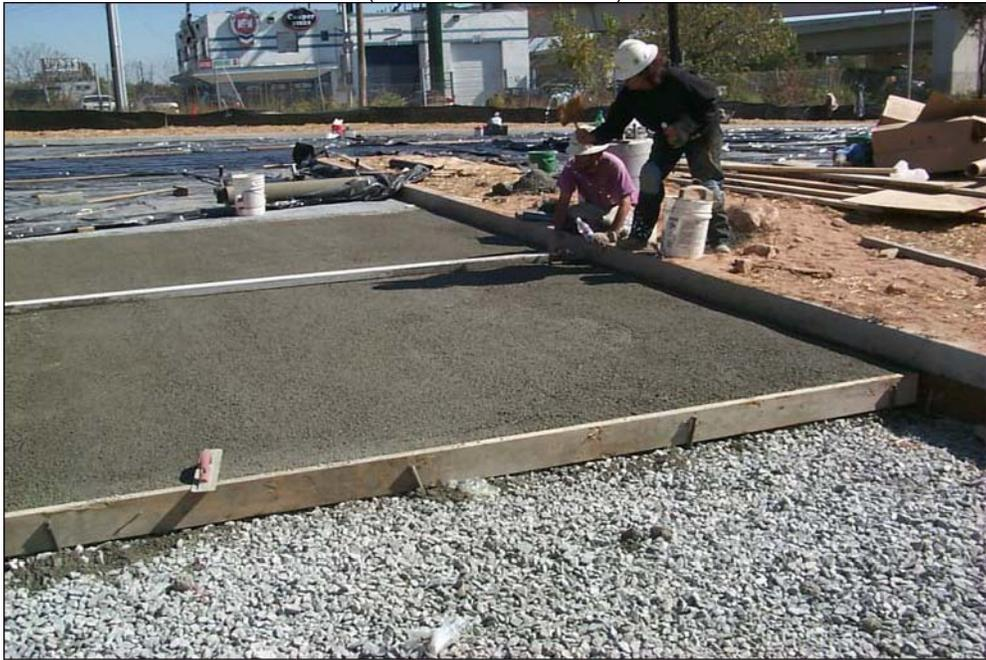
**Figure 2.2.24-2 Porous Concrete System Installation**
